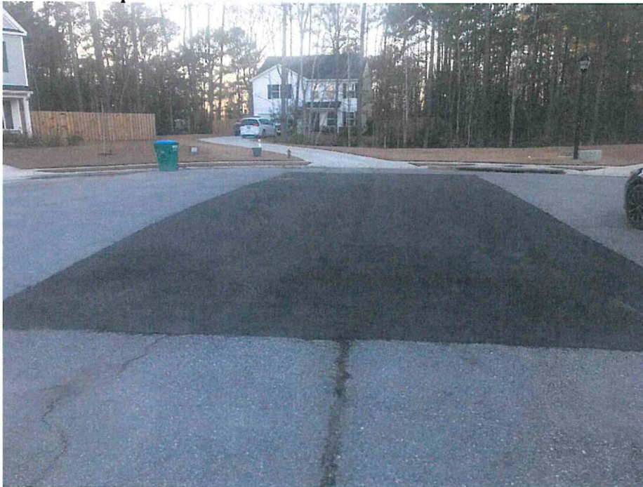
Pavement repair on Honeysuckle Court
