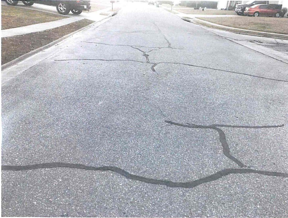
Crack sealing has been completed.
