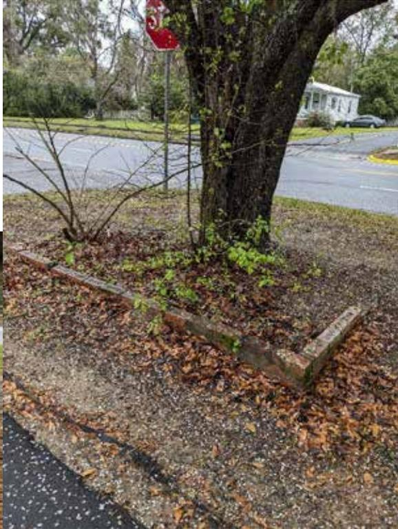
The brick boxes shown above are in a state of disrepair and should be removed. Plants in the planters should be removed as well, leaving the trees to match the rest of the trail. All bricks removed should be preserved to repair the existing planters by Guyton Elementary.
